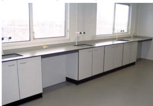
Perimeter benching fitted with sinks, taps and gas taps
