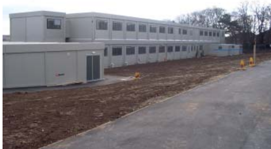
Multi storey modular buildings can be provided when space is at a premium
