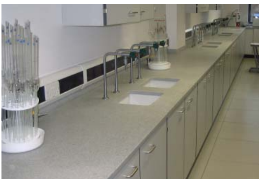
Perimeter benching with sink cut outs Sussex Coast College, Hastings
