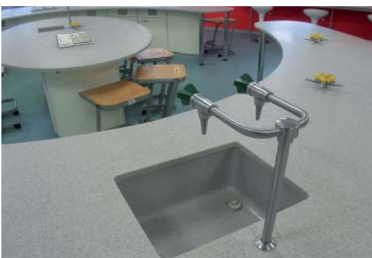
Sink cut out and elliptical island bench Dr Challoner's Grammar School, Bucks
