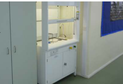
Fixed fume cupboard
