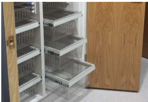
Corridor cupboards fitted with HTM71 cabinets
