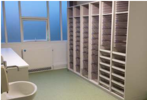
Clean utility room with HTM71 tall cabinets
